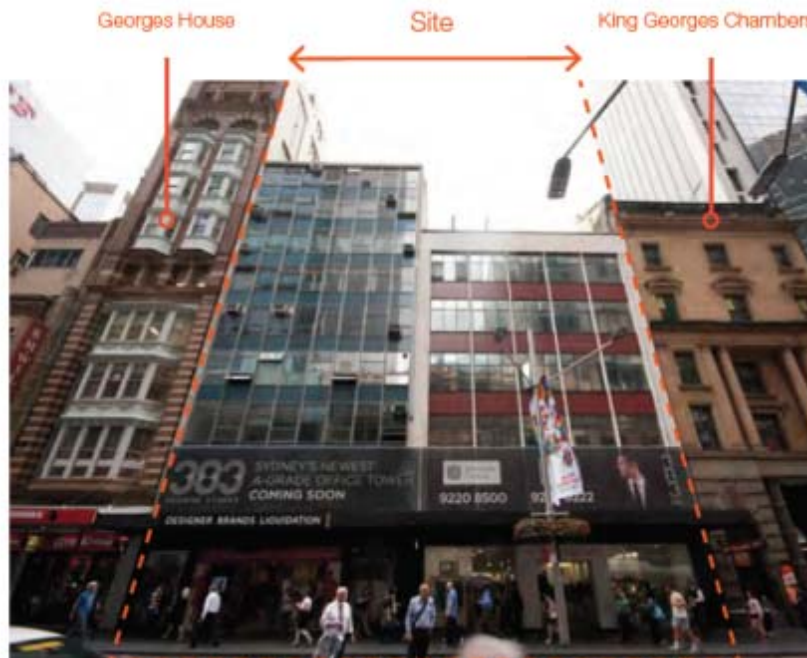
Figure 2: Site viewed from George Street (photo source: Mecone)
